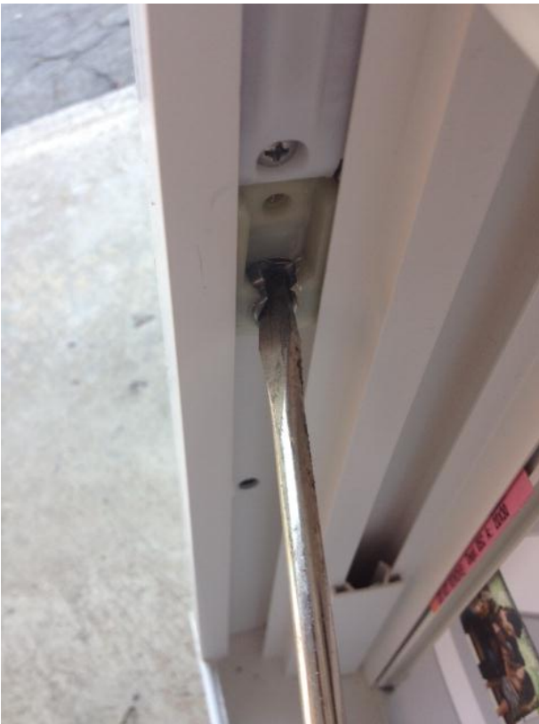
Spring disengaged
